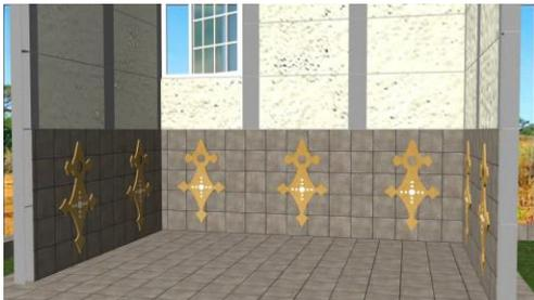
**Fig. 8. Floor and wall covering in M-DP panels**
